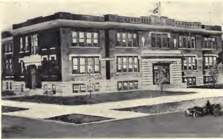
THE ROBINSON TOWNSHIP HIGH SCHOOL, ROBINSON, CRAWFORD COUNTY
